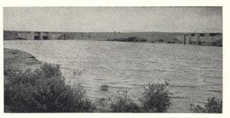
A view of the dikes and control structures in the Cheyenne Bottoms. The water, flowing into the area via the Wet Walnut inlet canal, is diverted through the control structure at the left into the main pool, where it will be impounded and used to flood the perimeter pools.
