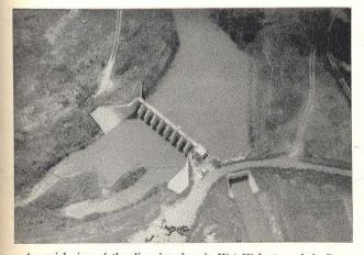
An aerial view of the diversion dam in Wet Walnut creek in Barton county. Flood waters may be seen being diverted through the control structure at the right into the inlet canal, thence on down into the Cheyene Bottoms proper.—*Photo courtesy Sharon Foster*.
